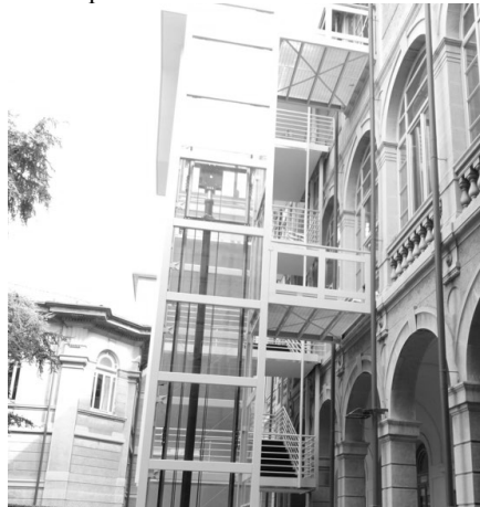
Fig. 1. Structural system for a steel elevator
