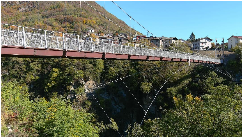
Fig. 1. Overview of the Suspended bridge above the Mallero river
