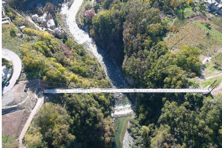
Fig. 14. Aerial view of the suspended bridges above the Mallero river
