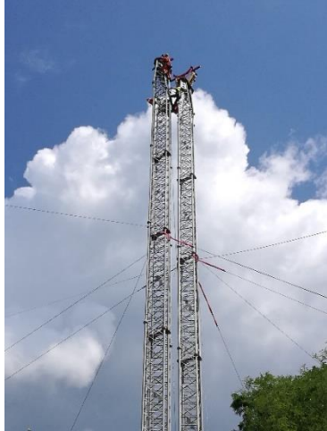
Fig. 9. Installation of the cableway
