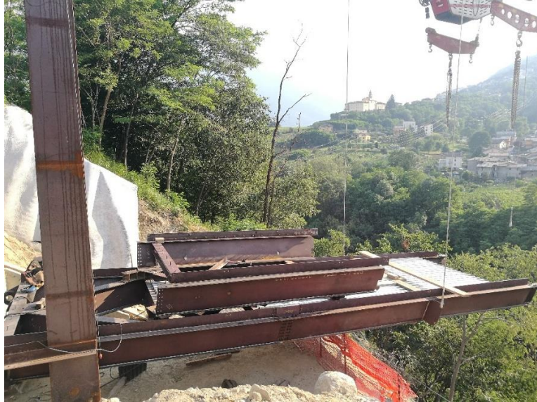
Fig. 12. Installation of the first pieces of the deck
