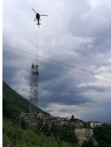
Fig. 10. Installation of the cableway
