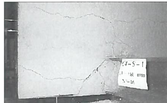
Fig. 5 Damage in the concrete slab.
