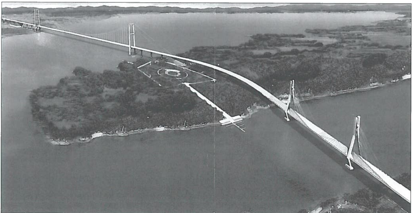
Artist's impression on the Runyang Bridge when completed in 2005. Suspension bridge on the left, cable-stayed bridge on the right. (Photo: Jiangsu Provincial Yangtze River Highway Bridge Construction Commanding Department)
