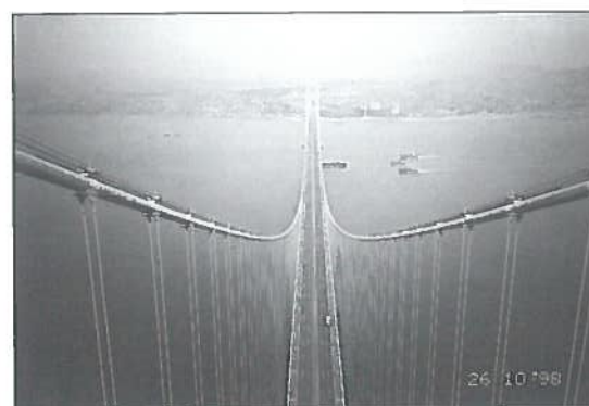
Akashi Bridge: view towards Honshu in the north (Kobe side). Photo taken at the top of the south tower (Awaji side). The north tower is looming in the background, at a distance of about 2 km. (Photo: Juhani Virola)
