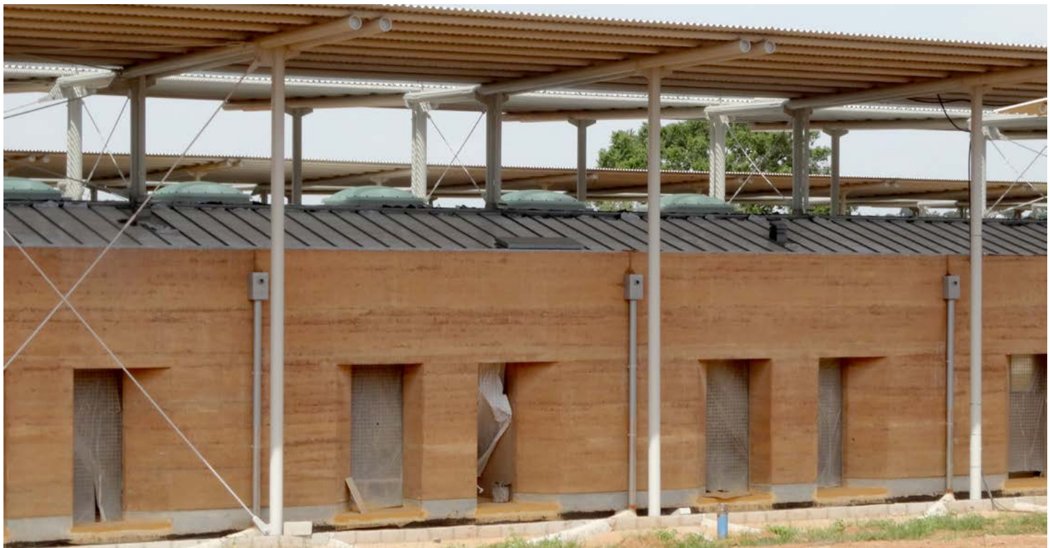
Fig. 48 – Vista dell'ala sud. © Emergency NGO Technical Department
