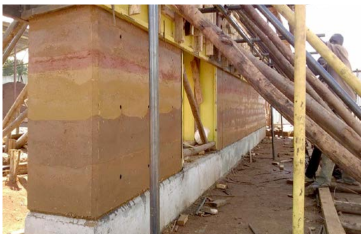
Fig.19– Dettaglio del mock up della muratura in pisé. © Emergency NGO Technical Department
